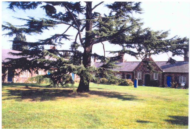
The view from the front of the site including the chapel.
