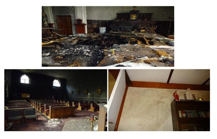
The fire, soot, smoke and extinguishment water damage within the church itself was substantial and smoke permeated into the presbytery which has resulted in further cleaning and decorating costs. The extinguishment of that one candle and the removal of combustible materials from its proximity would have avoided a claim that has run into hundreds of thousands of pounds.
